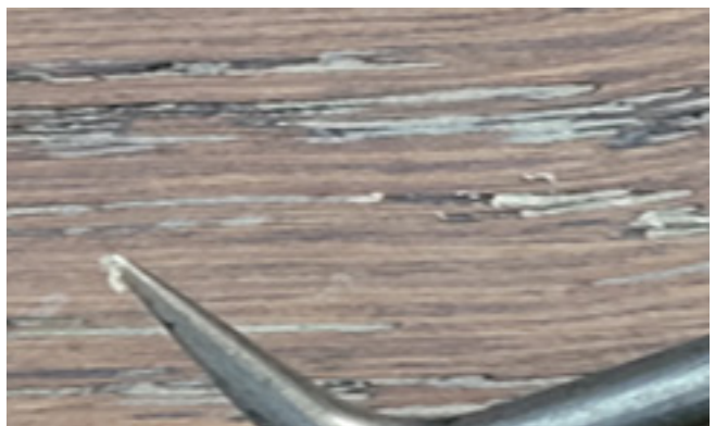
Drywall dust embedded in brushed surface Cause: Poor scheduling of work and/or lack of adequate floor protection
